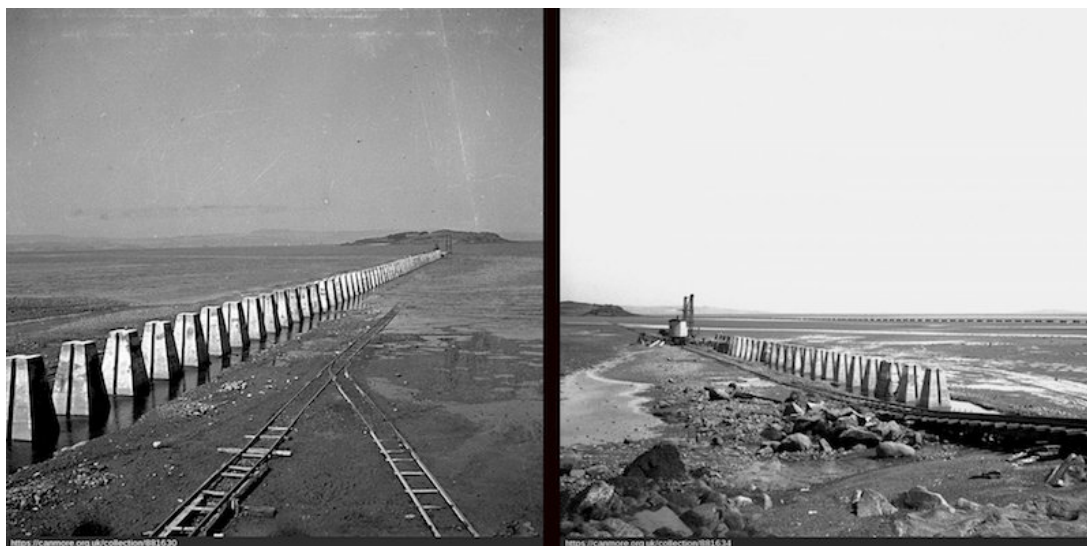
Views of the anti-shipping barrier running from Cramond to Cramond Island, showing construction work in various phases, 1940. Copyright Royal Commission on the Ancient and Historical Monuments of Scotland/Crown Copyright, OER
