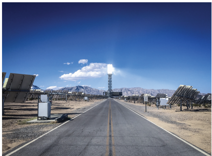
Fig. 4, Flashback to a daylight lantern, Ivanpah Solar Power Facility, Mojave Desert, California
